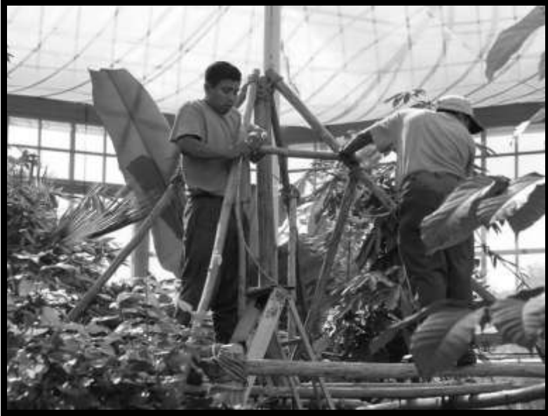
Beginning construction of the Maya House. Photo by Brendan Sayers
